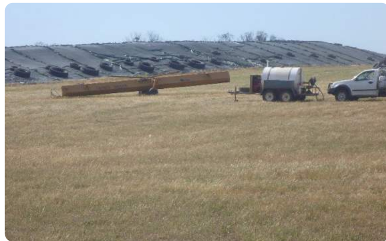
Figure 1. An example of an in paddock silage pit constructed of easily accessible materials such as black plastic and tyres as weights.
